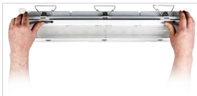
Reinstall diffuser
